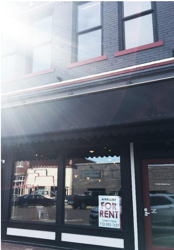
Figure 16 Mixed Use Building
